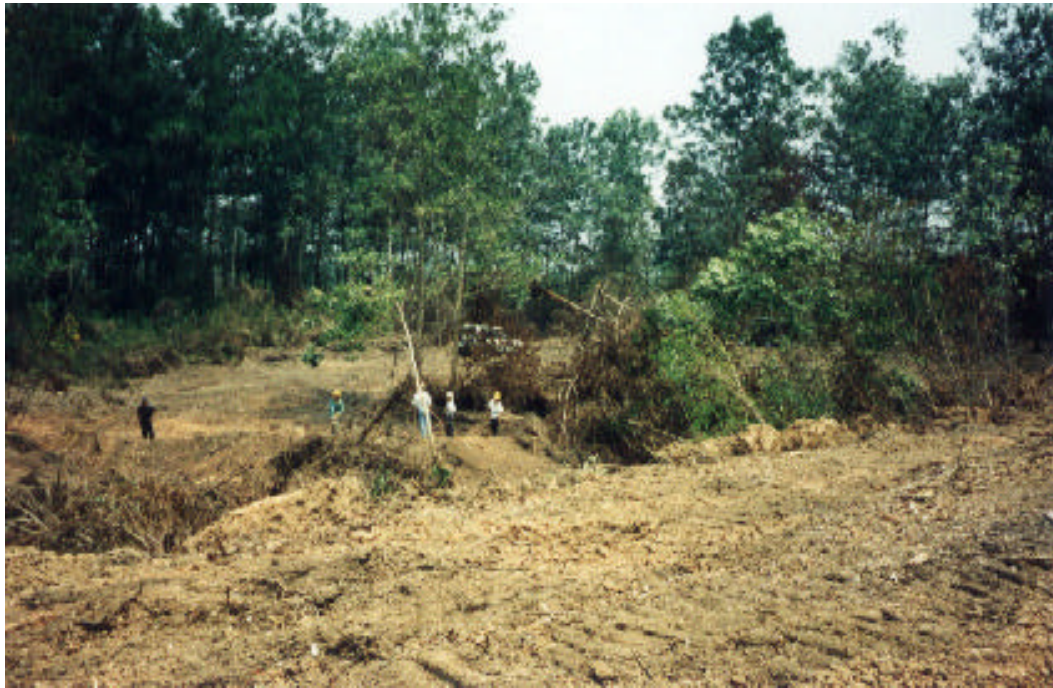
Plate 17. Bulldozer construction of a large firebreak; Suban Jeriji, August 1997.
