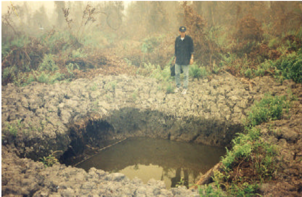
Plate 10. Hole dug to obtain a water supply for fire fighting in PT. Sribunian, October 1997.
