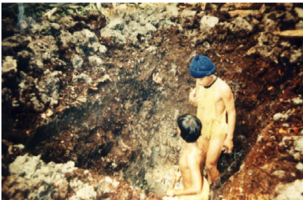
Plate 12. Digging a hole to obtain a water supply in PT. SBA Wood Industries, October 1997.
