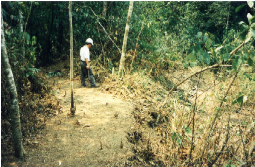
Plate 16. Construction of a bare-ground firebreak with hand tools; Suban Jeriji, August 1997.
