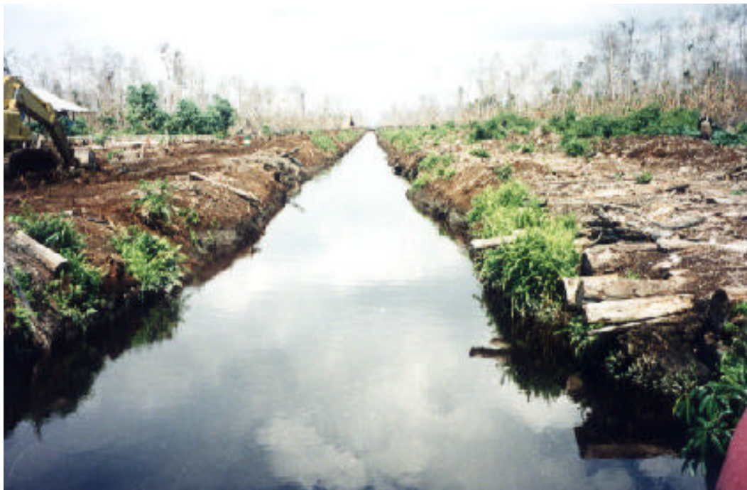
Plate 3. Canal used for commercial timber extraction in PT. SBA Wood Industries, Bina Hutan Base, March 1998.
