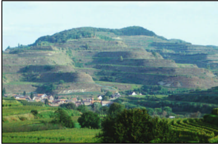
Fig.2. With the consolidation and restructuring of farmland in the 1960's and 70's, large terraces were constructed with slope heights stretching up to 40 m with over 100% inclination. Since their establishment they have been treated only in exceptional cases.
