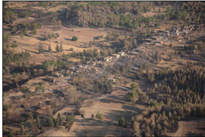
Figure 4. A village damaged by wildfire (Photo: OGM)
