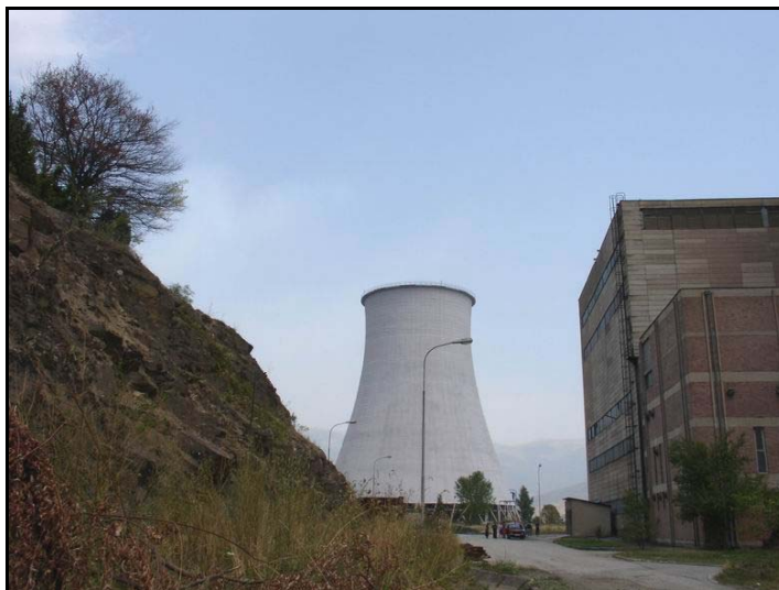
The electric power plant Oslomej near Kicevo was at threat to be affected by wildfires burning at the very edge of the facility (left in the photograph) by burning embers (spot fires) falling out on the structures of the power plant.
