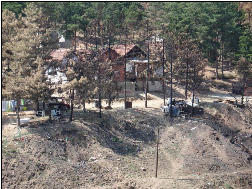
Fire-affected informal settlement of Roma at the outskirts of Bitola
