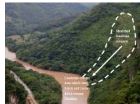
Landscape with indication of landslide (Photo: Geohazard expert team)
